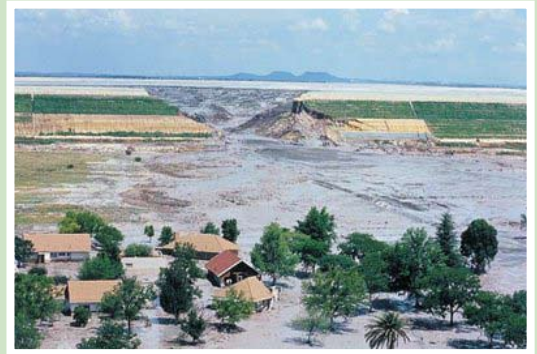
Image of the Merriespruit Tailings Dam failure in South Africa (image from Tailings.org)
